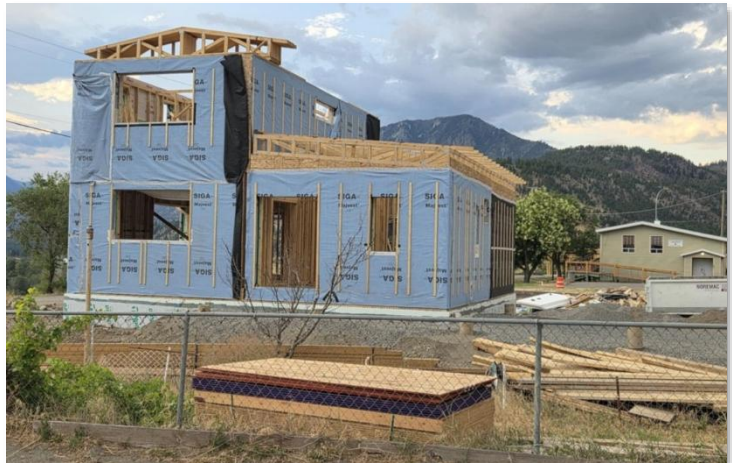
Rebuilding homes in Lytton
