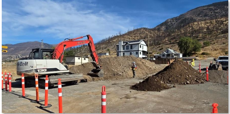
Village water system upgrades
