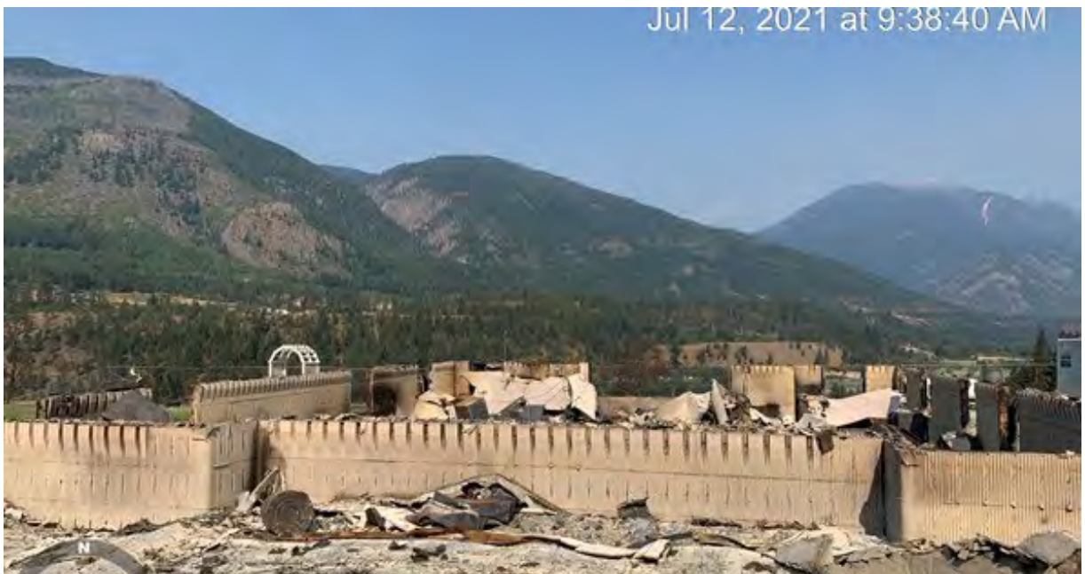
Photo 2 View of burnt structures | Facing west | July 12, 2021
