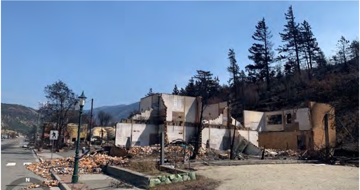
Photo 5 View of damaged building and hazardous goods | Facing northeast | July 15, 2021
