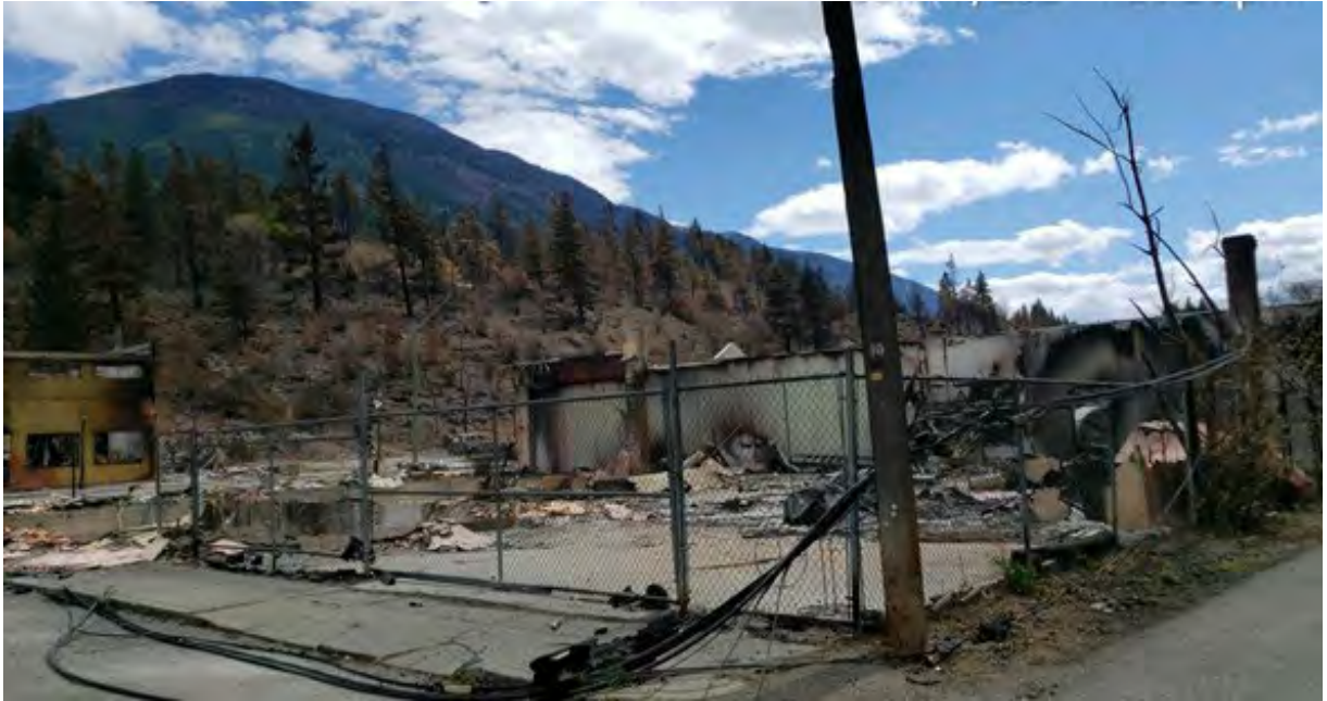
Photo 7 View of damaged building and hydro pole | Facing southeast | July 17, 2021
