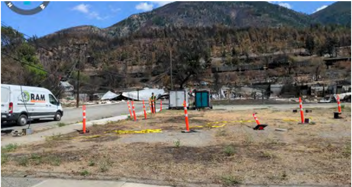
Photo 15 View of former hazardous materials stockpile area in Zone 3A | Facing southeast | July 22, 2021
