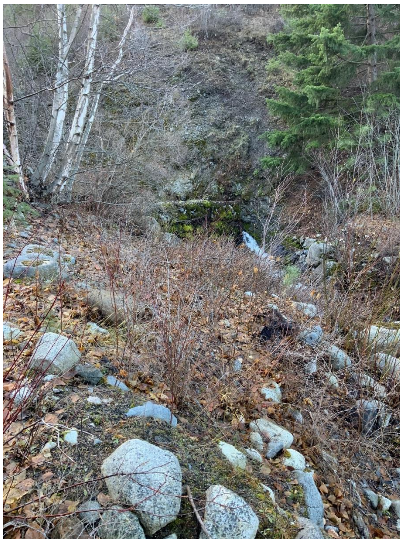
The dam for the In Stream Reservoir
