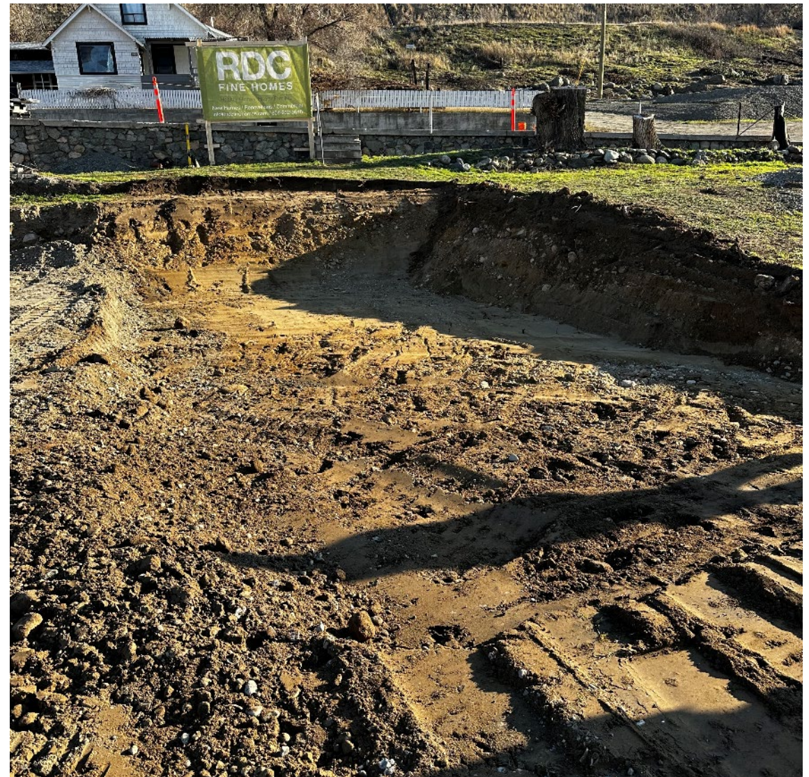
Excavated portion for new basement
