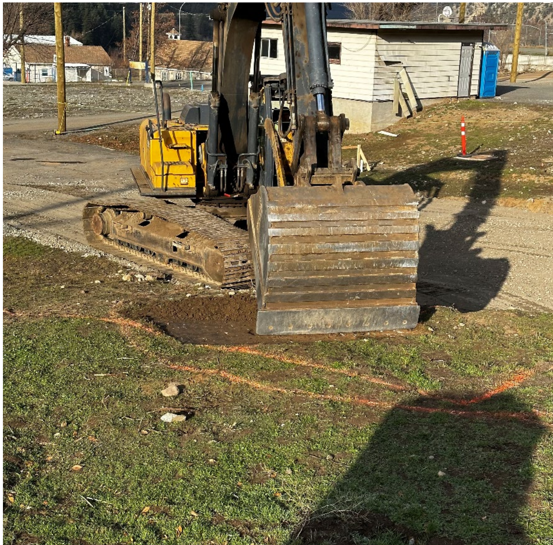
Start of excavation – removing soil with potential cultural material carefully
