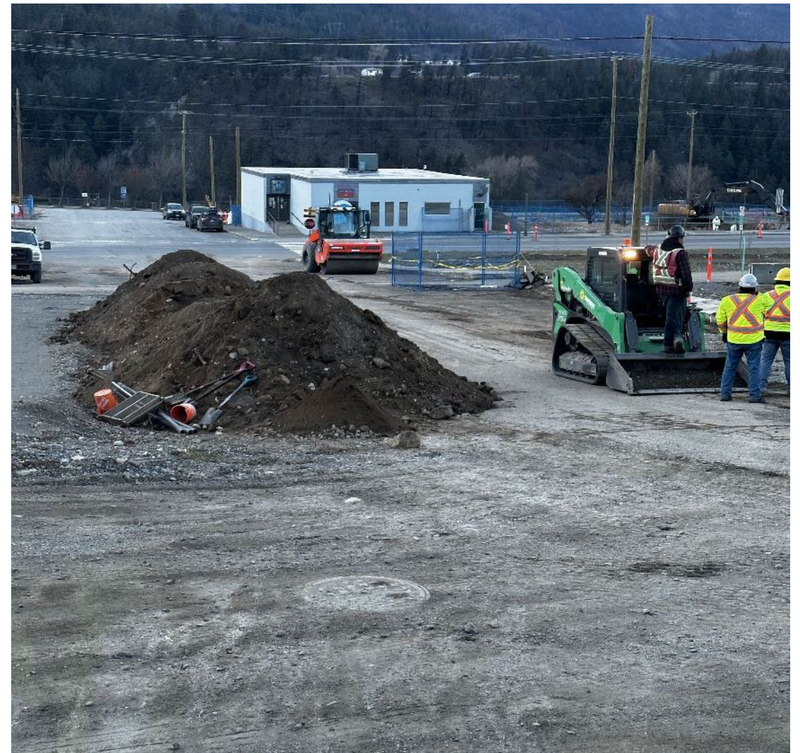
Removed soil being sifted
