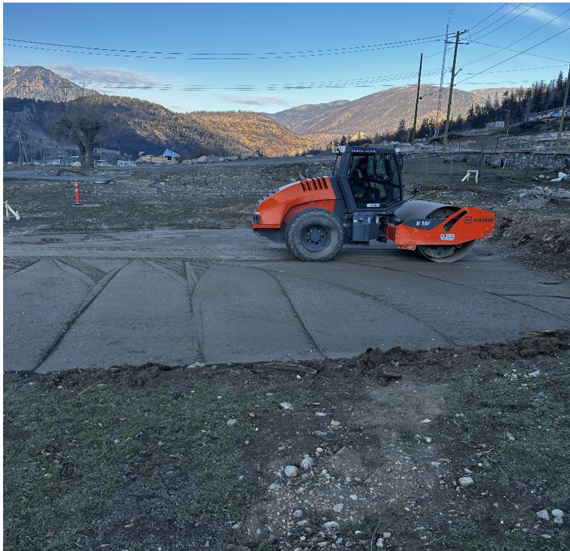
Compactor preparing fill for foundation
